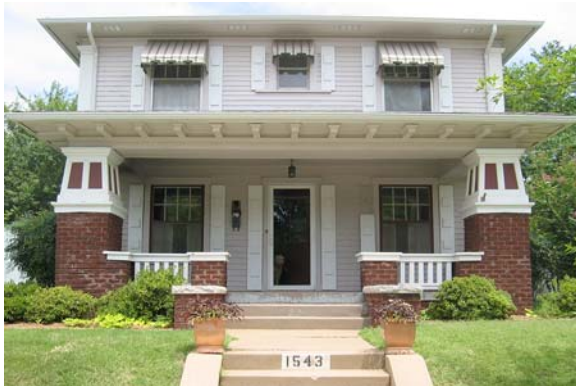
A.7.2 Two examples of inappropriate shutters. Neither house style would have originally had shutters. On the left, the shutters aren't half the width of the window, so they don't appear operable. Also, door shutters are completely inappropriate. On the right, grouped windows wouldn't be flanked by shutters.
