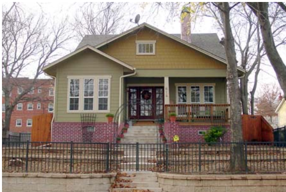
C.1.1 / C.1.2 While not a duplicate of existing houses, this house draws upon common characteristics of the district – raised crawl space, porch design, multiple front gables, siding patterns and grouped windows.
