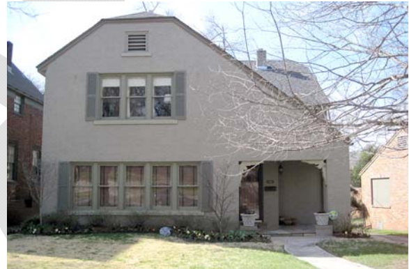
A.7.2 Two examples of inappropriate shutters. Neither house style would have originally had shutters. On the left, the shutters aren't half the width of the window, so they don't appear operable. Also, door shutters are completely inappropriate. On the right, grouped windows wouldn't be flanked by shutters.
