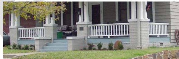
Traditional design with railing lower than piers.
